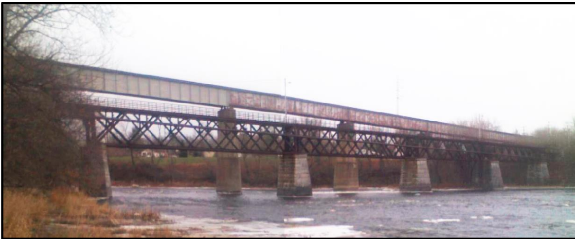
Massena rail bridges crossing the Grasse River, truss bridge in foreground, girder bridge in background
