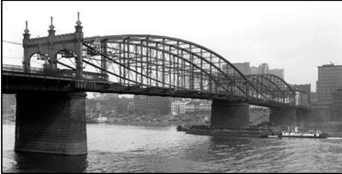
The Smithfield Street bridge in Pittsburgh, Pennsylvania, looking from upstream in 1933 [1]
