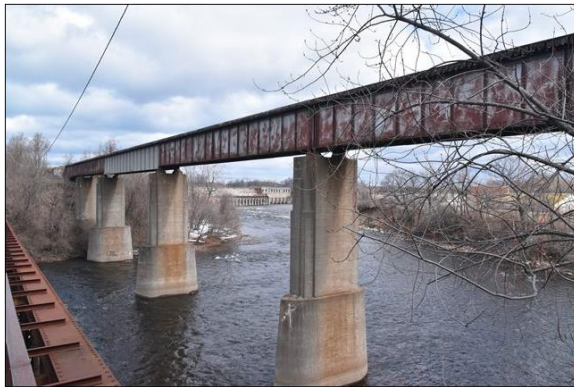
MTRR Girder Bridge over Grasse River [1]
